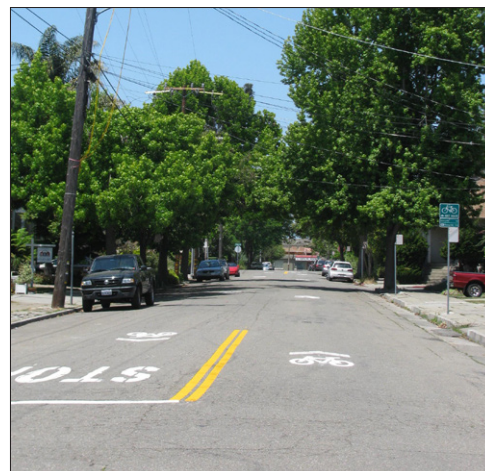
Figure 5: 50 ft double centerline
